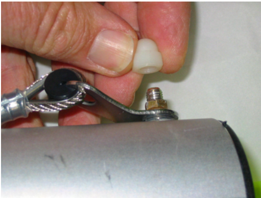
Installation of clinch nut
